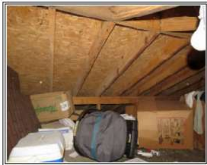
Head & Shoulders View of Attic
