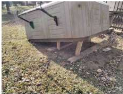
MPR-Safety hazard / Sauna not secured or
